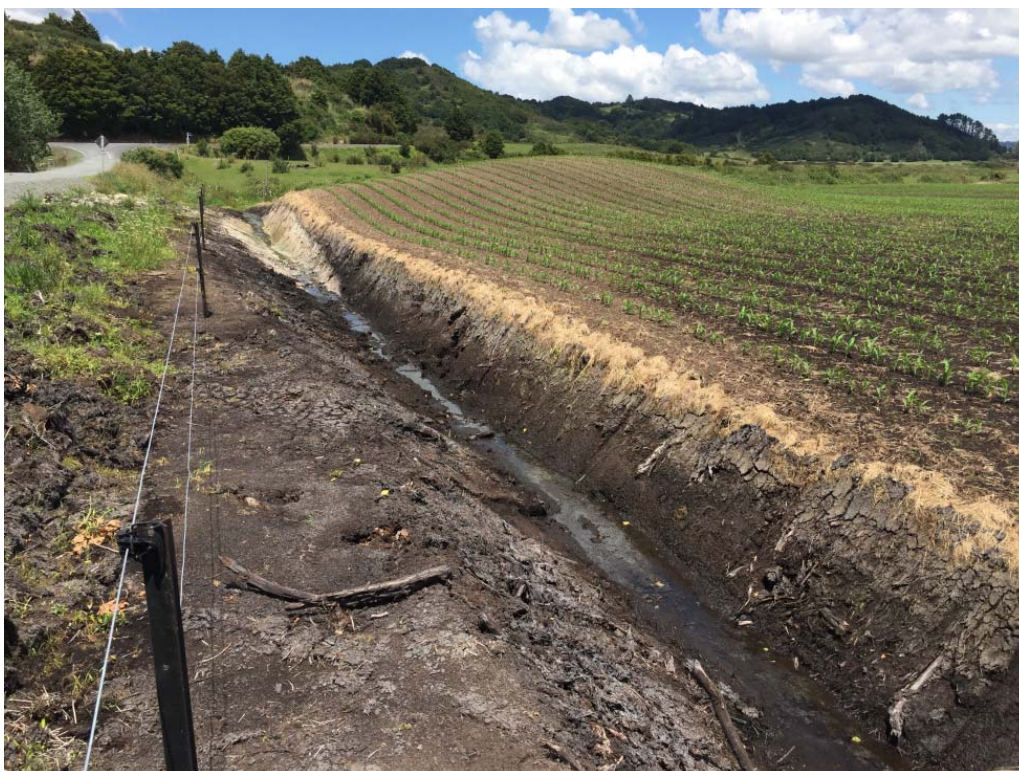
Figure 7 Drained peatland growing maize alongside Riponui Road, near the intersection with Heaton Road. The recently excavated drain shows a cross-section through peat, with a clay mound further along the drain forming the substrate under the low hill. This peatland was once continuous with Otakairangi.
