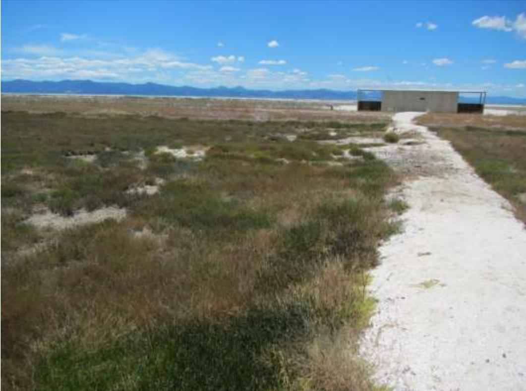
Plate 11: MNT bird watching hide (Unit 2). Scoured-out section of raised path should be replaced by boardwalk to allow unimpeded tidal flows.
