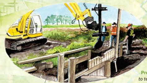
Peak run-off control structures are being trialled in the Carran Creek catchment where small dam-like structures are built in drains to temporarily pond water, providing more time for contaminants to drop out before being carried downstream, and lessen the intensity of flows to reduce bank erosion.
