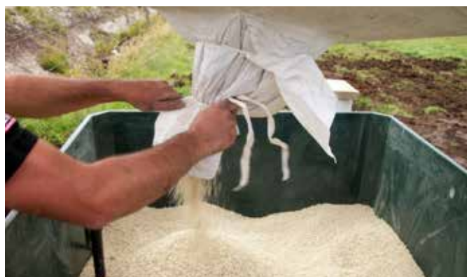
Phosphorous passive filter installed on private land. Aluminised zeolite will help remove phosphates from tile drains prior to entering into waterways.
