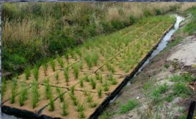
Floating wetland at Lake Areare inlet to improve water quality by reducing nutrients in surface water before it enters the lake (in collaboration with NZTA).
