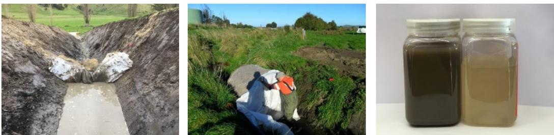
*Figure 23: Temporary hay bale and geofabric sediment filters and upstream / downstream water samples*
